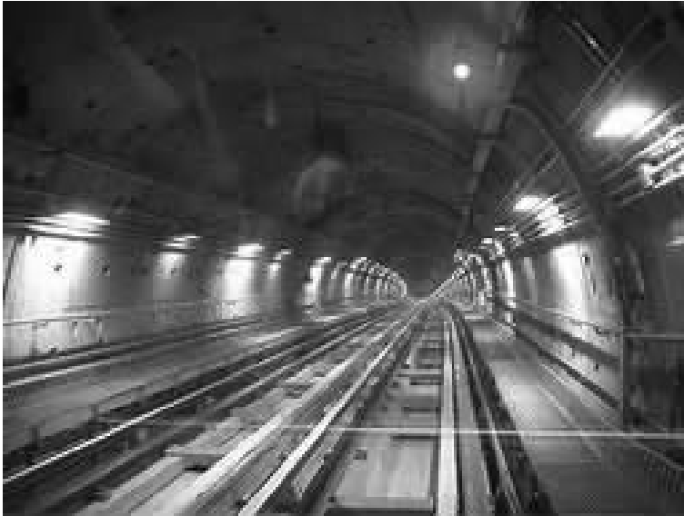
Figure 1.2 A Metro Tunnel
